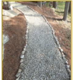
Infiltration Path - a trench filled with crushed stone that traps stormwater. Can replace dirt paths susceptible to runoff.
