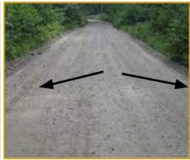
Crowning - A dirt road must be slightly pitched so water will run off of it instead of forming potholes and gullies. The high point can be in the middle to direct water in both directions, or on a far side to direct all water in one direction.
