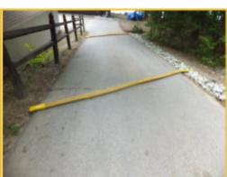
Firehose Diverter - In paved driveways, burying rubber and wood are not an option. Old firehose, or other durable material, can be filled with sand or stone and placed on an angle to divert stormwater. These have the added benefit of being movable.
