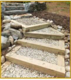
Infiltration Steps - Crushed stone steps that trap stormwater instead of allowing it to flow downhill.
