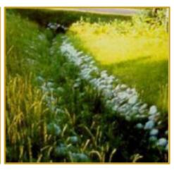
Ditching - Once water is directed off the road, it should flow into a pervious ditch to allow it to infiltrate. There are various methods such as vegetation and check dams which can be used to slow stormwater down in a ditch.
