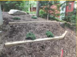
Water Bars - 6"x 6" lumber is installed on a slope with crushed stone on the uphill side to trap and divert stormwater. Water bars are left slightly raised to slow water down an can be used as seen above, or placed in a pathway in shorter lengths to function as steps.
